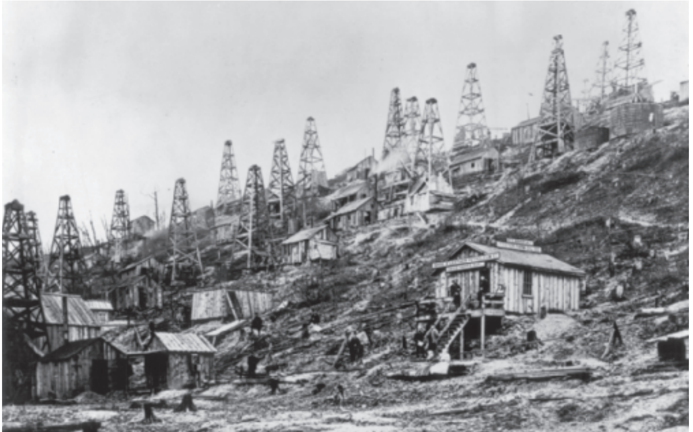
PIONEER OIL RUN, 1865 The American oil industry emerged first in western Pennsylvania, where speculators built makeshift facilities almost overnight. An oil field on the other side of the hill depicted here had been producing 600 barrels a day, and the wells quickly spilled over the hill and down the slope shown in this photograph. ( Library of Congress )
