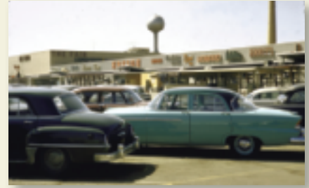
SHOPPING CENTER, NORTHERN VIRGINIA This small shopping center near Washington, D.C., was characteristic of the new “strip malls” that were emerging in the 1950s to serve suburban customers who traveled almost entirely by automobile. (Charles Fenno Jacobs/ Time Life Pictures/Getty Images )
